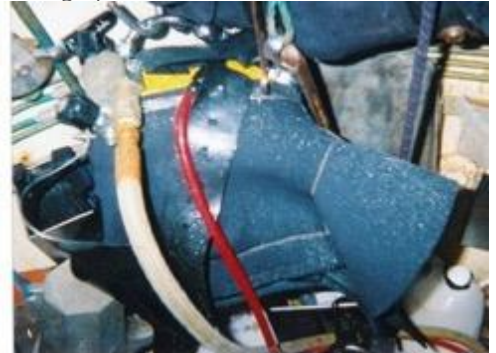
CO 2 dust on bellman's breathing equipment below scrubber
