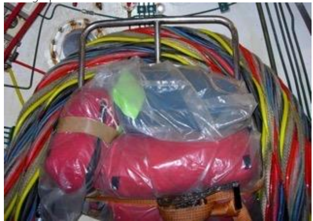
Typical storage of SPs 1 & 2 within a bell
