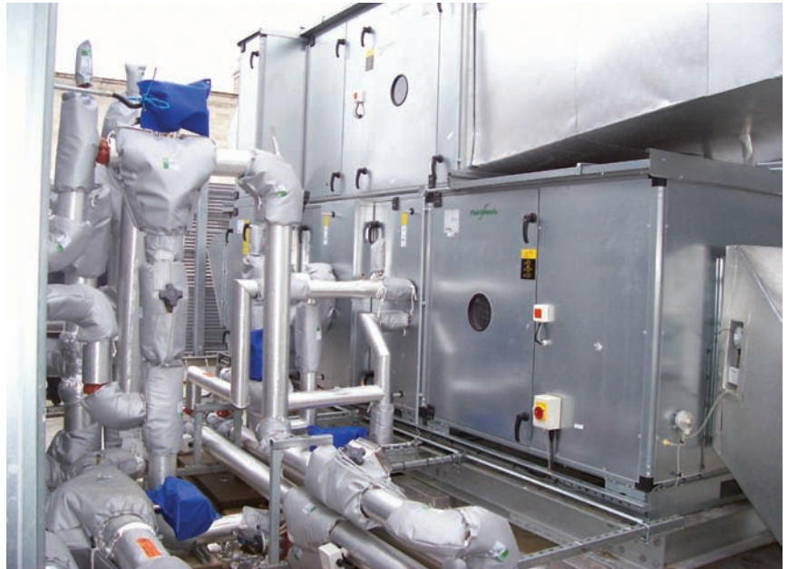
The legacy of poor design: this air-handling equipment was mounted double-stacked on the roof. Owing to the associated pipe work, safe access to the equipment within the units was not possible as there was no space for either a scaffold to be erected, or ladder to be positioned correctly. A double-decked access gantry has since been retrofitted.
