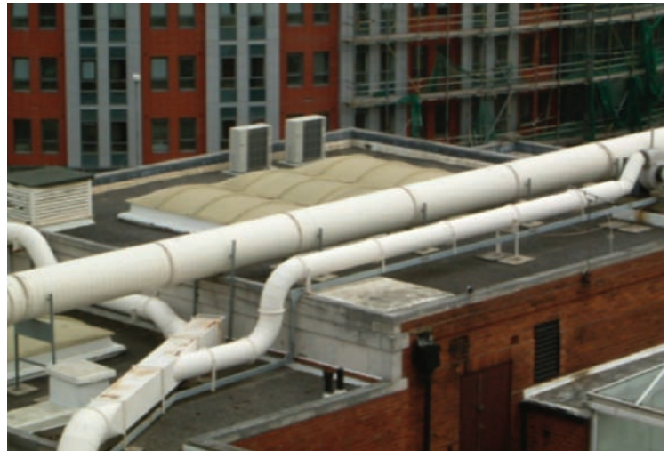
The legacy of poor design – the initial location of these condenser units precluded safe access for maintenance. They have since been relocated.
