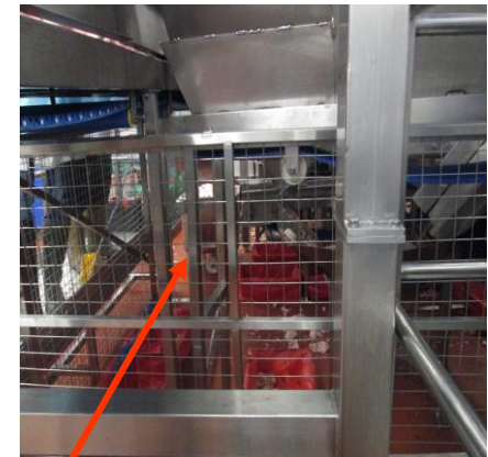
New Infill Panels Near Operators
