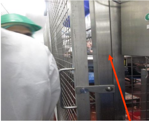
New Sliding Gate with Interlock
